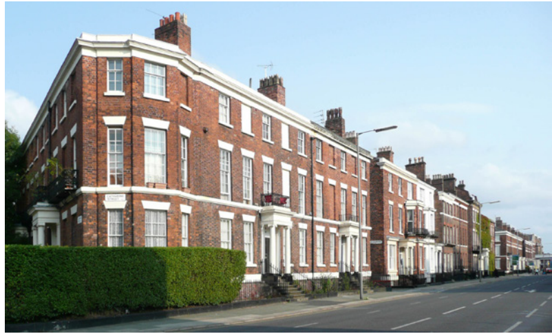
1864,4. The east side of Catharine Street from Canning Street to Upper Parliament Street in 2014. GHJ.
