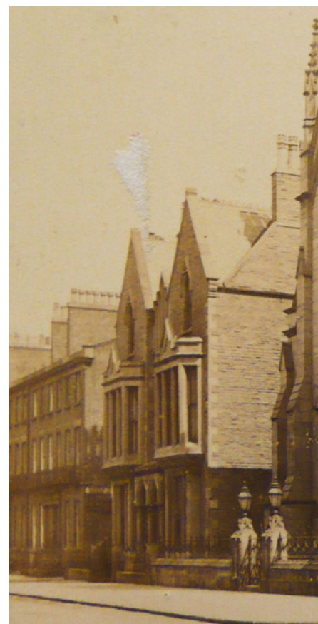
1864,32. A detail from the late 19th century photograph (from fig. 1864,18) showing the original design of the bay window parapets. LRO.
