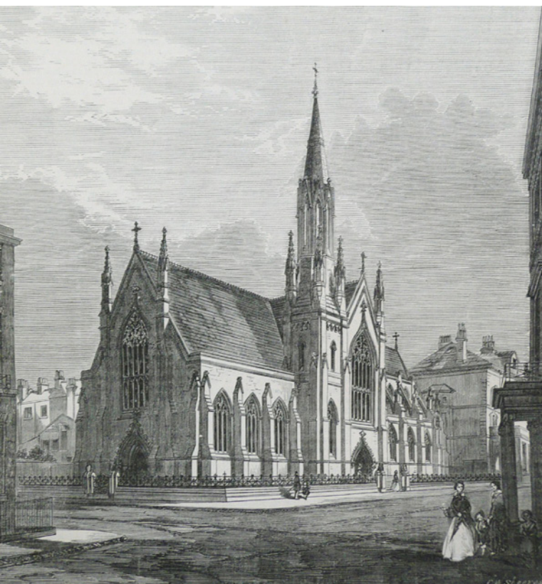
1864,5. The Catholic Apostolic Church (from a woodcut illustration in The Builder , 1857, p. 135). The building to its right is part of Napier Terrace in Canning Street; to its left is a view beyond the garden of 23 Catherine St to the rear of properties on St Bride Street (see fig. 1864,2). LCL.
