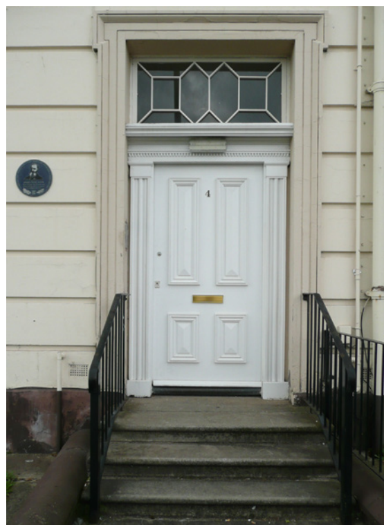
1833,10. The approach to no. 4 Clare Terrace showing the plaque on the wall to the left of the doorway. GHJ.
