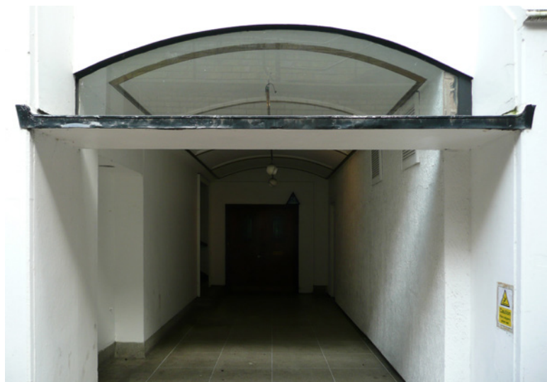
1989,7. All that is left of the entrance to the Oriel Restaurant viewed from Oriel Close in 2014. Immediately to the left of the scene is the dividing line between the building which survived the 1941 blitz and the new building by James and Bywaters which took its place (for a Covent Garden view of the old and the new see Footsteps , p. 207, fig. 12,4).
