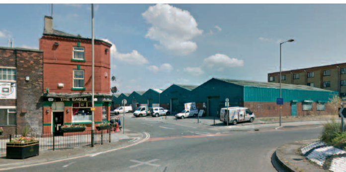
Blackstock Street/junction with Vauxhall Road, 2018. The Eagle pub is virtually the only survivor from 1900. The blue sheds mark where Blackstock Street Gardens once stood. Courtesy Google Street View.
