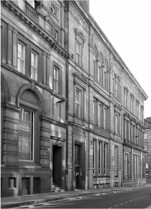
No. 5 Fenwick Street as it exists today, with its entrance in the centre of the view. Like several of the buildings in the area, following internal conversion it now provides apartments for those who enjoy living in the city centre.
